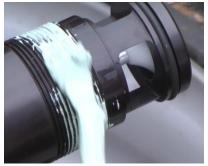
Figure 11-3 Apply Thread Sealant
